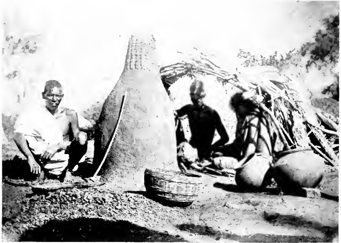
Fig. 24. Pariahs smelting small "blooms" of wrought iron, Salem district.
